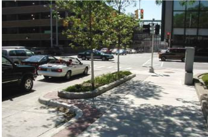
Example of Curb Extension or Bulb-out
